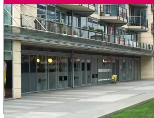
Commodore House Battersea Reach, SW18 Client: Private Investor
