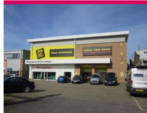
5-7, Weir Road Balham, SW12 Client: Private Company
