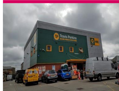
2-6, Weir Road Balham, SW12 Client: Private Landlord
