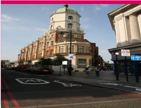
Toplin House Brixton, SW9 Client: Private Company
