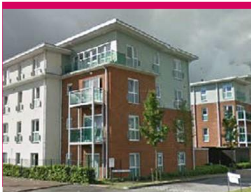
Former BMW garage Tunbridge Wells, Kent Client: Linden Homes, South East Ltd.
