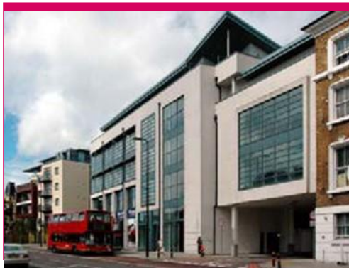
Former Savoy Laundry site Clapham Road, SW9 Client: Persimmon Homes Plc
