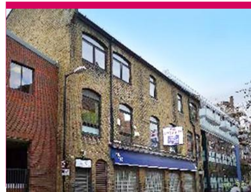
Rushworth Street London, SE1 Client: Mazeford Developments
