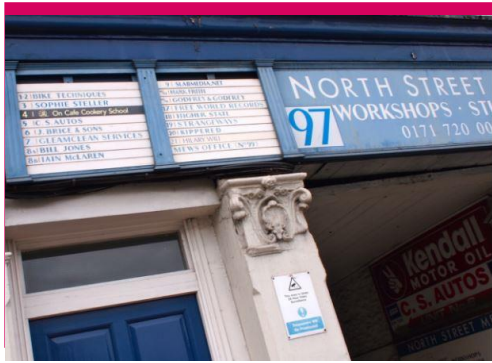
North Street Mews Battersea, SW4 Client: Highlaw Ltd
