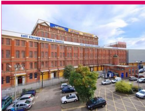
Ingate Place Battersea, SW8 Client: Safestore
