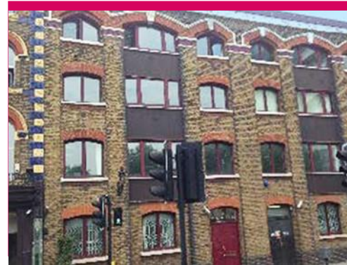
Albert Embankment Vauxhall, SW8 Client: OCUBIS Ltd.
