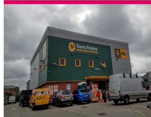
2-6, Weir Road Balham, SW12 Client: Private Landlord
