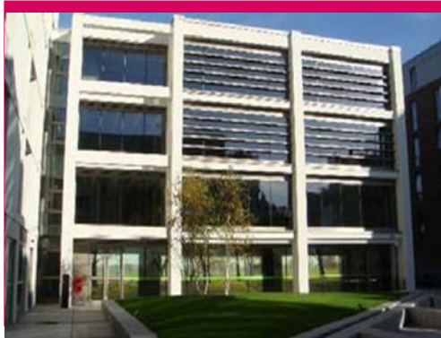
Wingate Square Clapham, SW4 Client: IPSUS Ltd.
