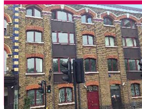
Albert Embankment Vauxhall, SW8 Client: OCUBIS Ltd.
