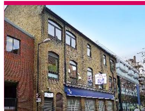
Rushworth Street London, SE1 Client: Mazeford Developments
