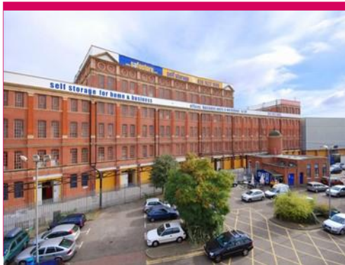
Ingate Place Battersea, SW8 Client: Safestore
